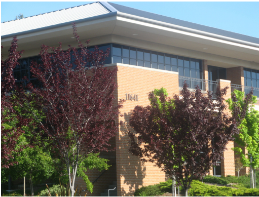
TCS Headquarters in Auburn California
